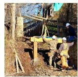
Work is well underway to replace the water wheel and the flume. This is essential for grinding to resume which is planned for May 2, depending on weather and pandemic protocols.
